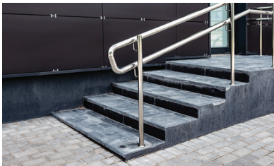
Staircases & its Metal railings
