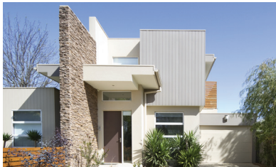
Vertical cladding of Stones
